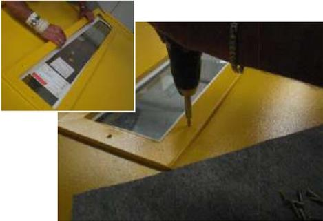
11.- Drill holes at the remaining fixing points and screw in the ring, **taking care not to over-tighten so as not to damage the glass.**
